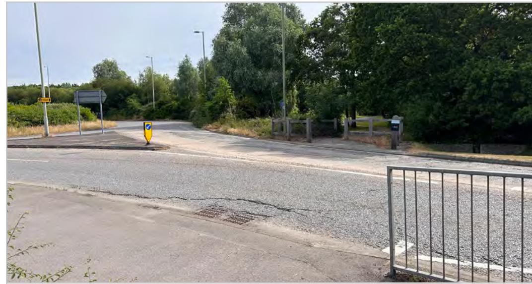
Z3.4.3 – Approach to Whiteley Way roundabout
