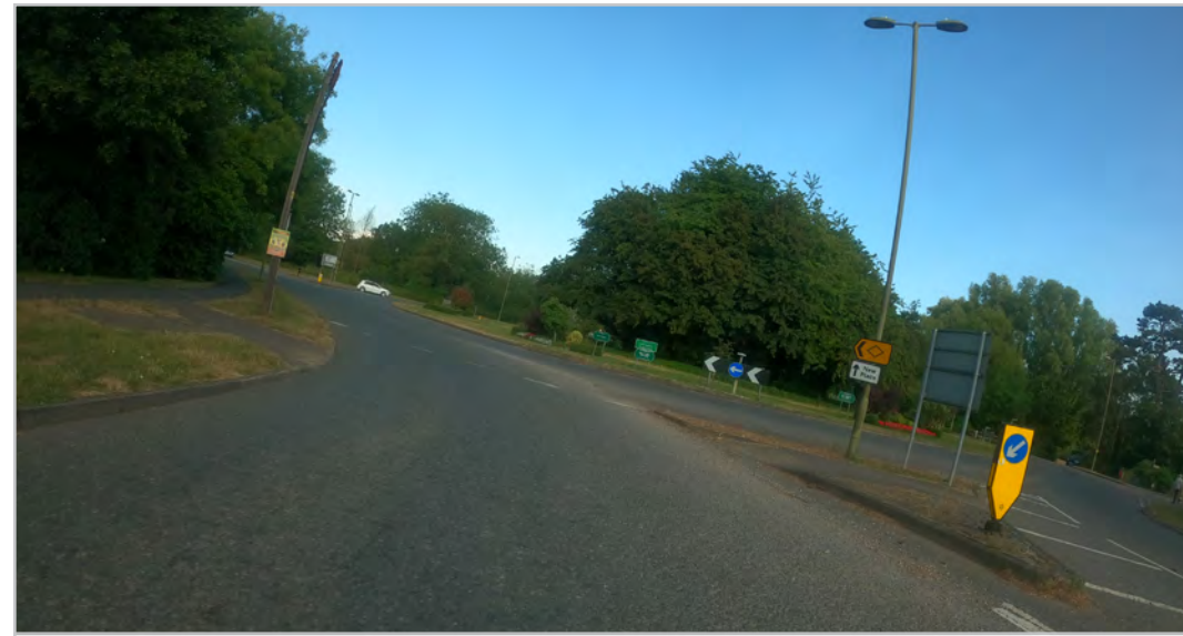
130.3.1 – Botley Road roundabout
