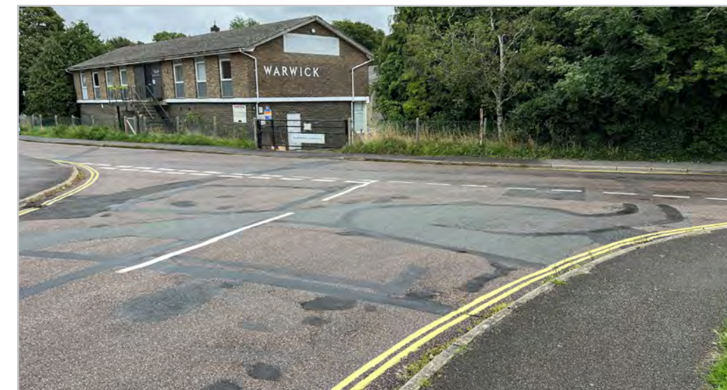
Z4.2.2 – Station Road/Buddens Road junction
