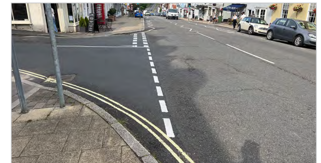
Z1.1.4 – West Street/Station Road junction
