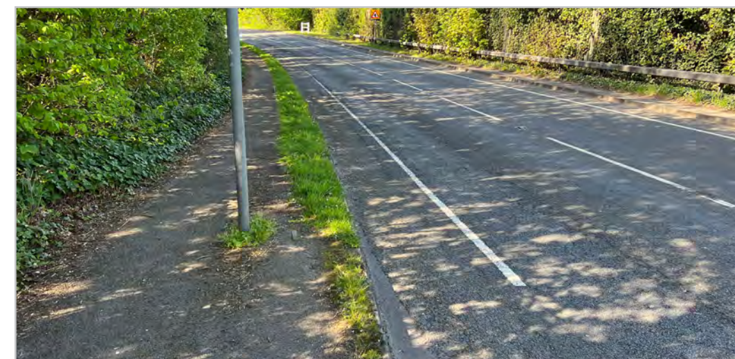
120.1.5 – Otterbourne Road between the motorway bridge and Southdown Road
