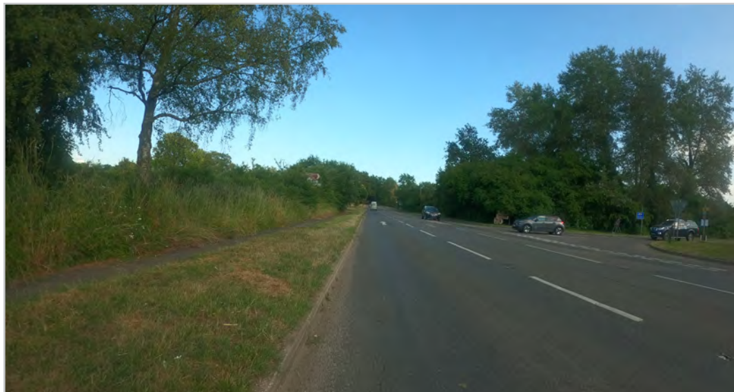
130.2.3b – Winchester Road / Winters Hill junction
