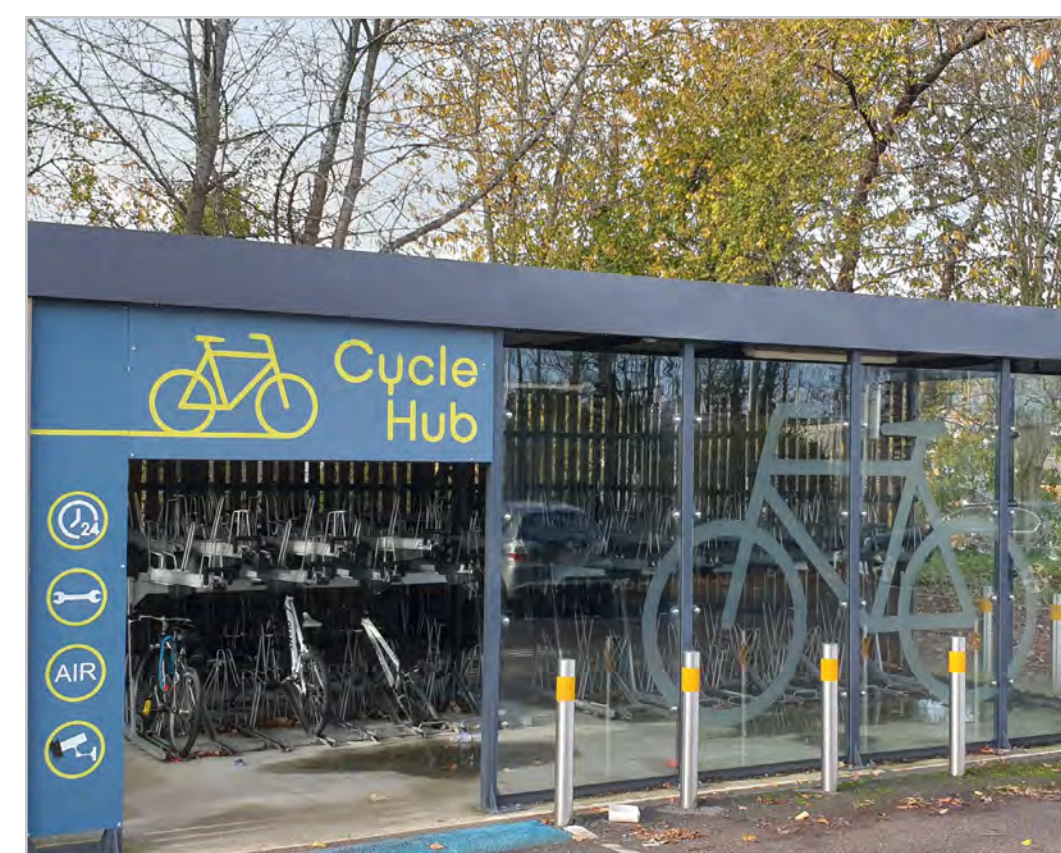
An example of cycle hub parking facilities – Winchester Train Station
