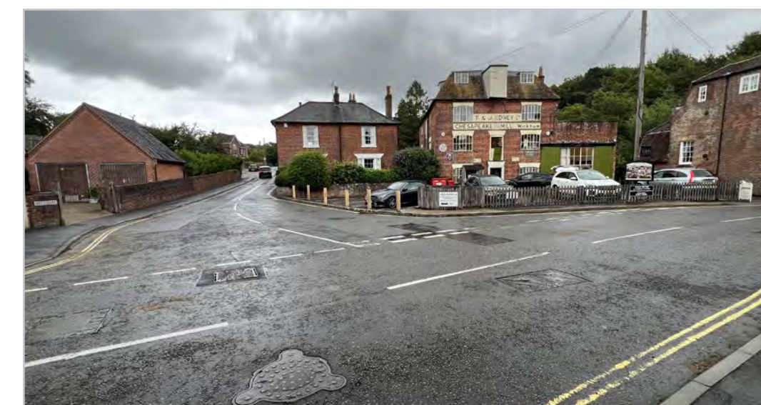
Z4.3.4 – Mill Lane/Bridge Street junction
