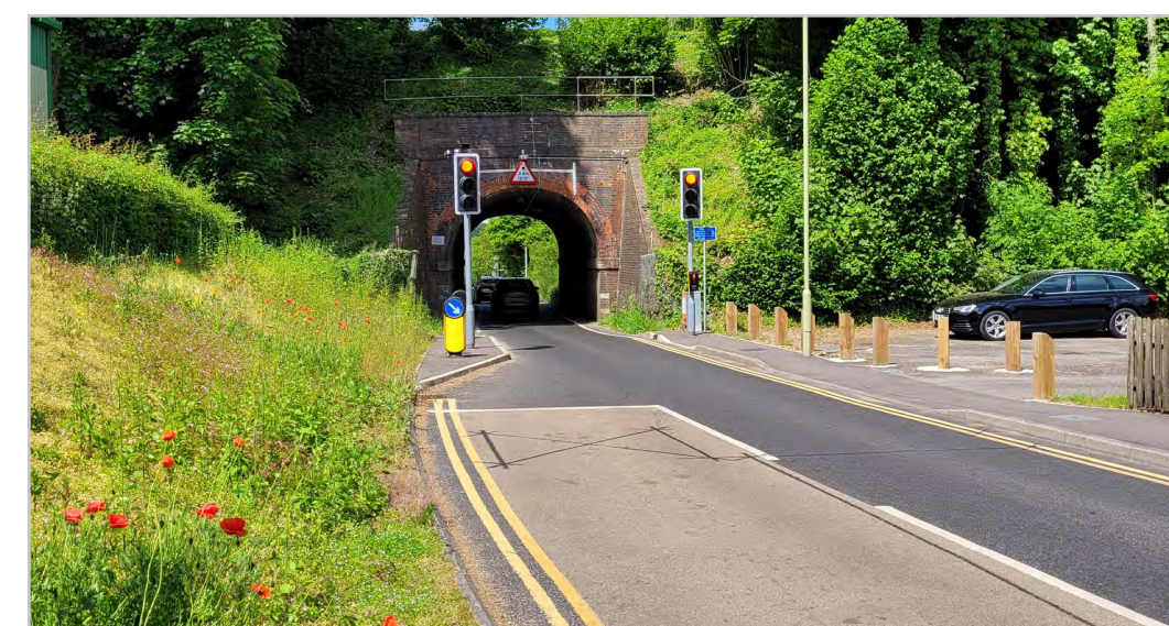
200.2.5 – Wellhouse Lane underbridge
