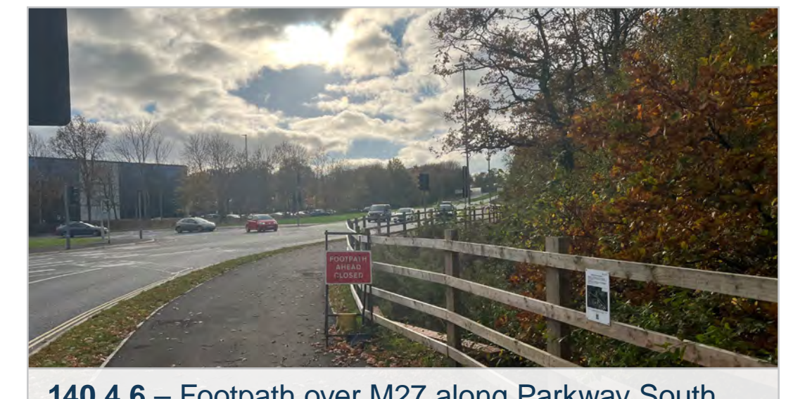
140.4.6 – Footpath over M27 along Parkway South roundabout
