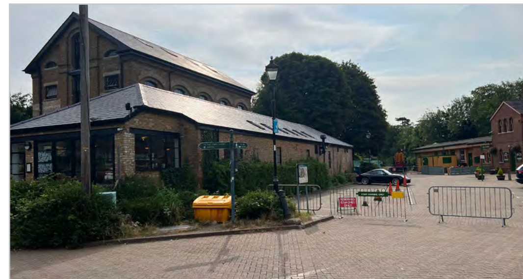
Z1.3.2 – New Alresford Railway Station car park
