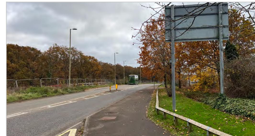
140.4.2 – Whiteley Way along Whiteley village
