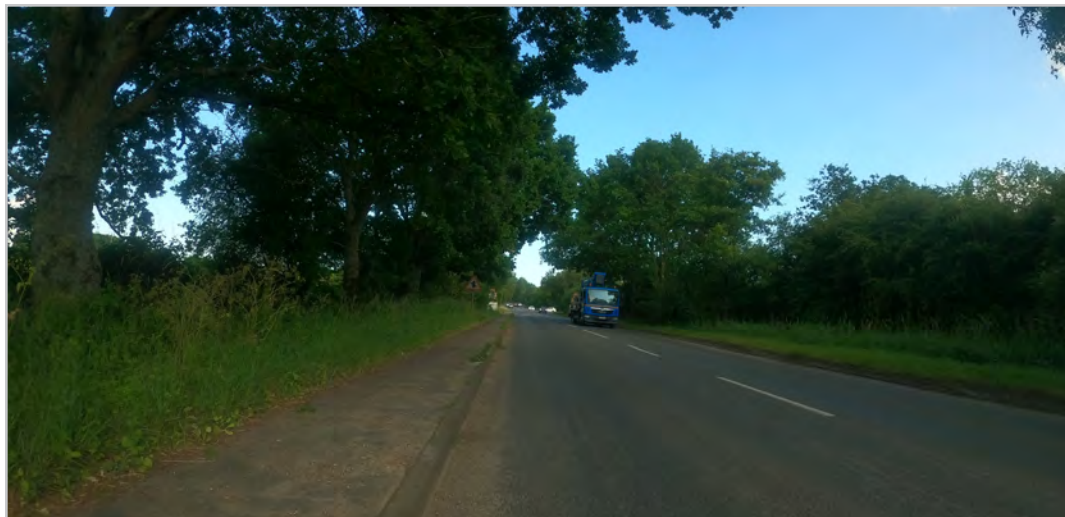
130.2.3a – B2177 between Lower Upham and Albany Road
