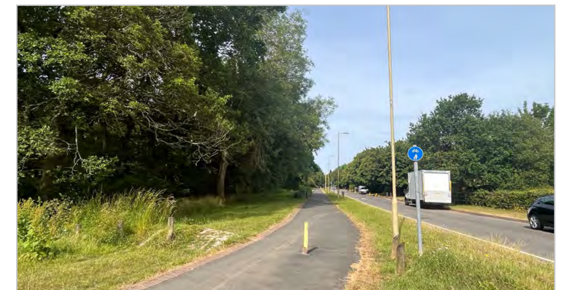
Z3.1.1 – Existing shared use path along Marjoram Way
