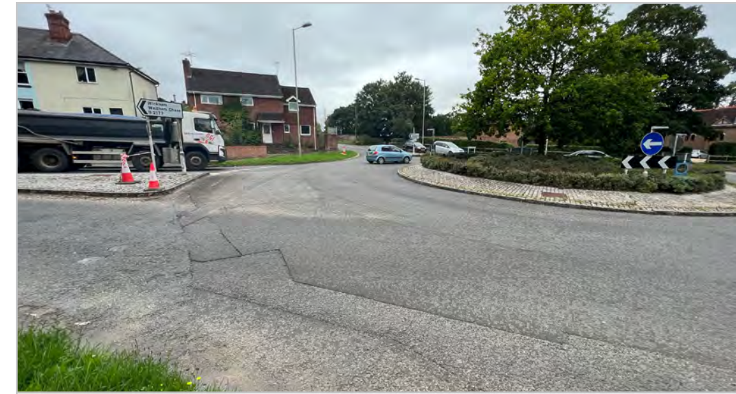
Z2.2.4 – B2177/Botley Road roundabout
