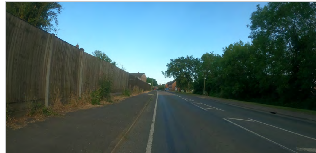
130.2.4 – B2177 between Albany Road and the B3035 roundabout
