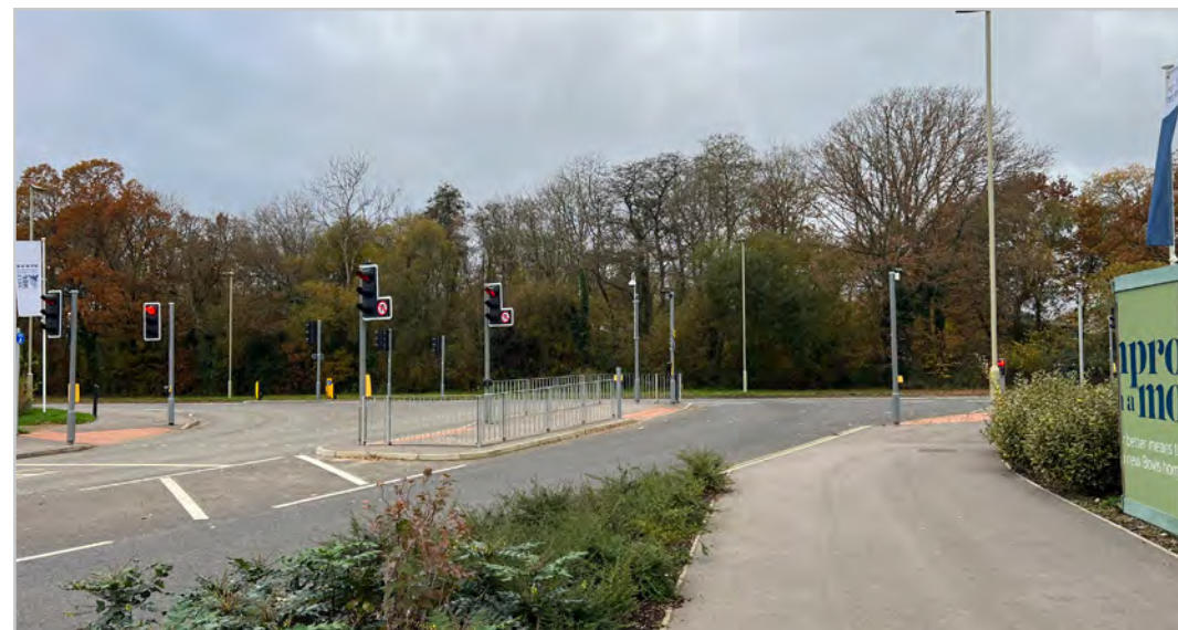
140.2.2 – A3051/ Whiteley Way Junction
