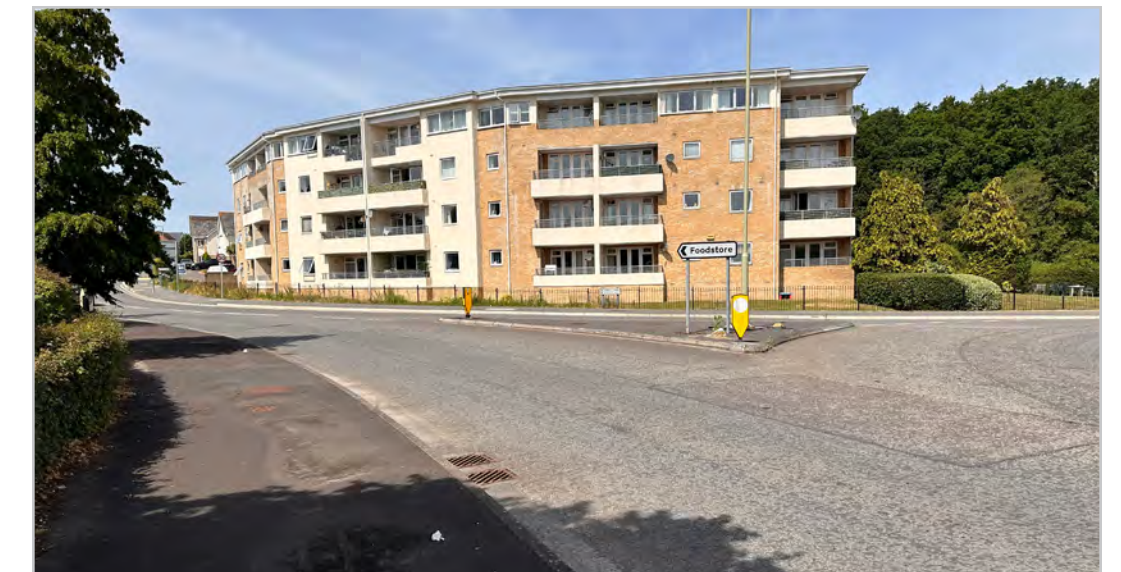
Z3.5.1 – Bluebell Way just off Whiteley Farm roundabout
