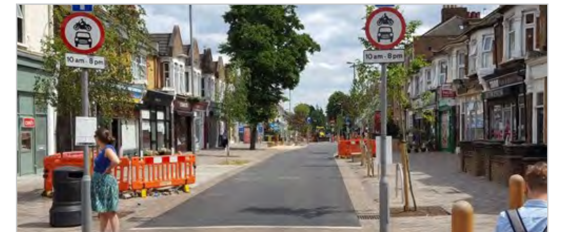
Francis Road, Leyton – Time restrictions on through motorised traffic, footway widening and bollards to allow for seating areas
