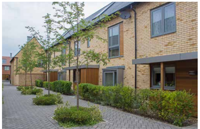
Above: Streets should offer an attractive environment, and not be orientated around vehicles (Trumpington Meadows, Cambridge)
