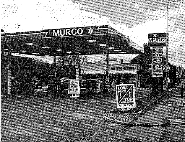
Poor example of over signage providing visual clutter.
