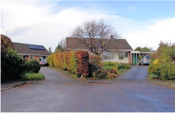
Figure 19: Cul-de-sac mid-20th century bungalows, Littleton.
