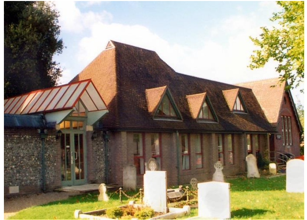
The Paterson Centre attached to the village church – sympathetically designed to match the original Victorian school schoolroom at the far end of the building
