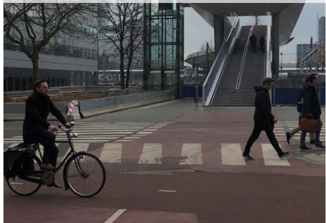
Figure 10.55: Cycle lift and wheeling ramps, Utrecht Station – most people use the ramps on the stairs because they are quicker but the lift meets the needs of people who cannot use them. (Note that the road markings do not comply with UK regulations.)
