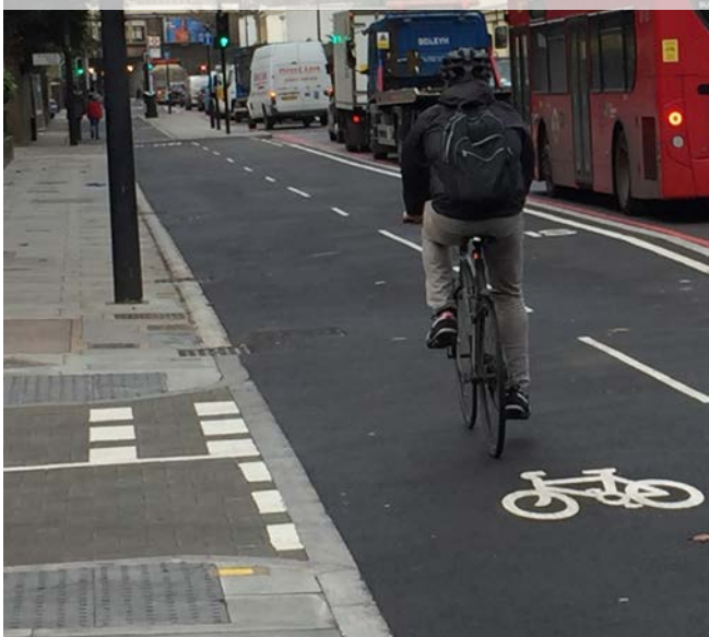
Figure 7.10: Tight kerb radii at residential side street
