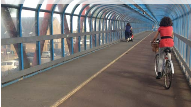
Figure 10.50: Covered pedestrian/cycle bridge across railway tracks, Cambridge
