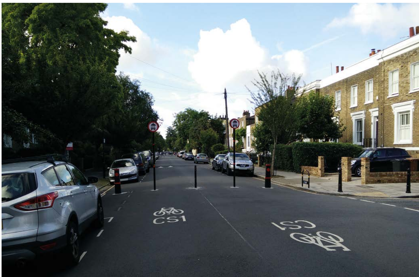
Figure 3.6: Simple mode filters, such as this one in Hackney, help form cycle-friendly neighbourhoods
