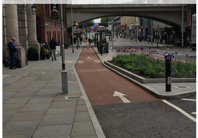
Figure 9.4: Cycle lane to cycle track transition
