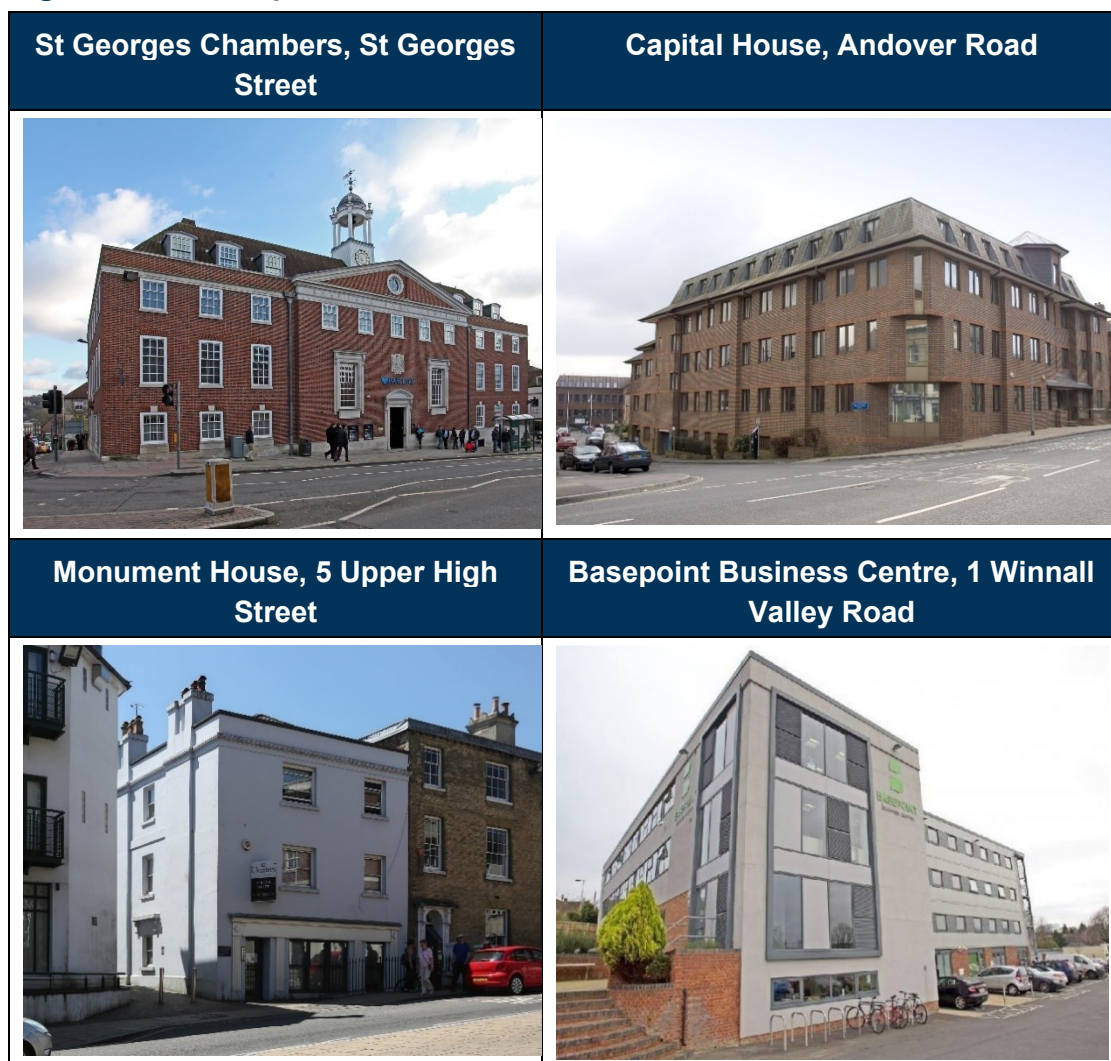
Figure 4.14 Examples of office units, Winchester Town
