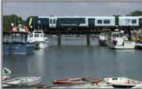
A South Western Railway train crossing the Lynton River, where work will include improving the durability of the wrought iron columns which support the viaduct
