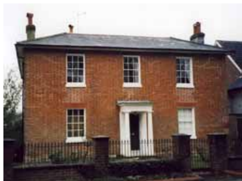
Bourne House from the Georgian era
