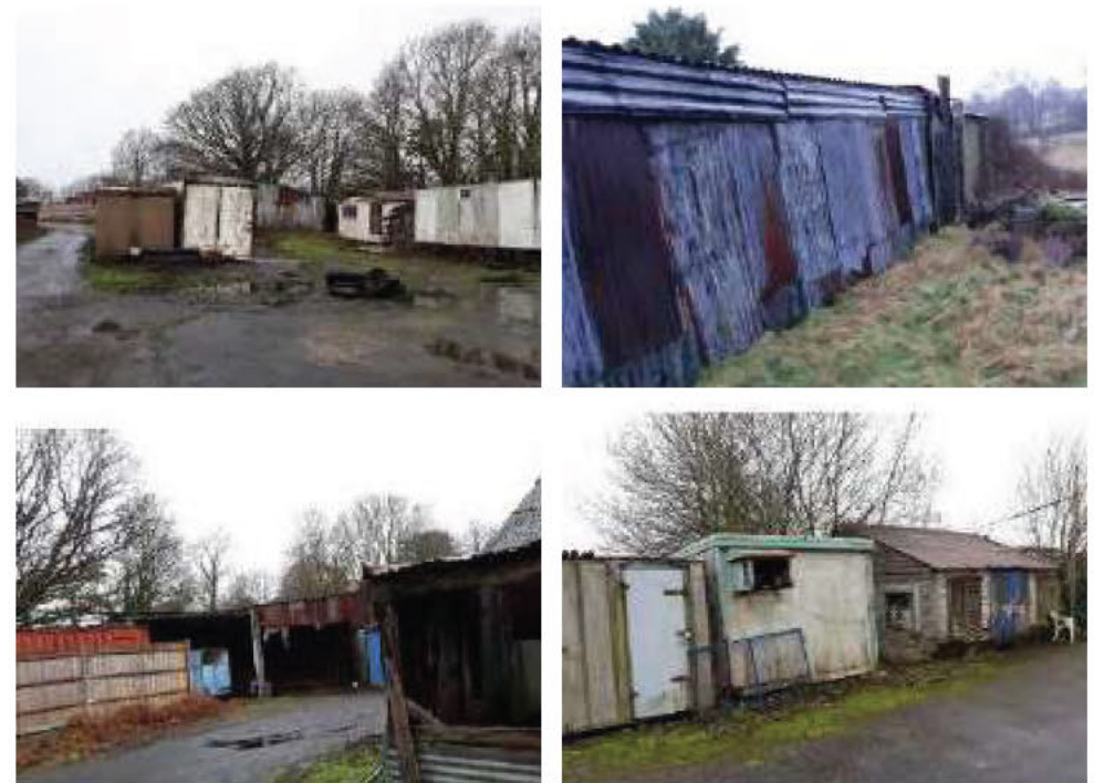
Figure 20: Existing site photos presenting derelict buildings.
