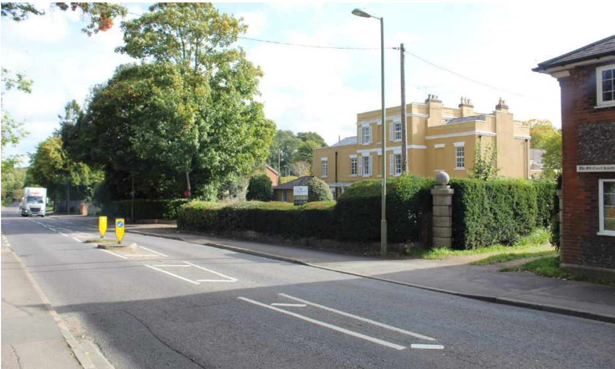
Image EDP 16: Typical view of Otterbourne House Grade II listed building, looking north-east along Main Street and illustrating its current setting.
