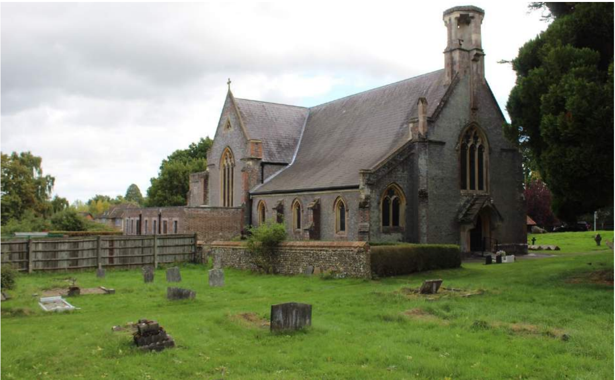
Image EDP 19: Typical view of the Grade II* listed Church of St. Matthew, looking north-east and showing the key aspects of its special interest.
