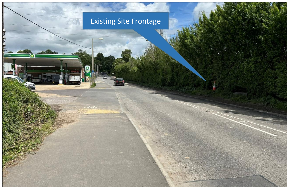
Figure 2.2: A334 Station Hill (Looking North)
