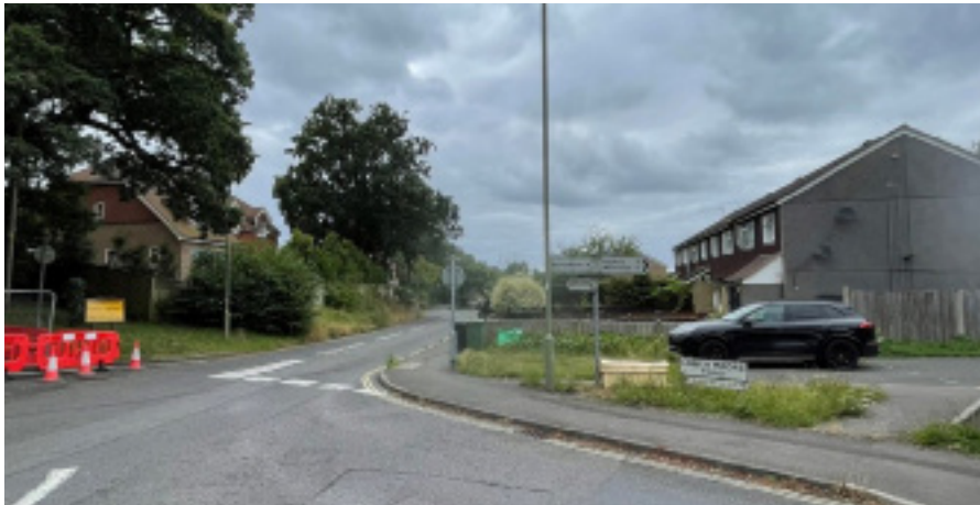
Figure 19. View towards northern boundary of Site from junction of Upper Moors Road and Spring Lane
