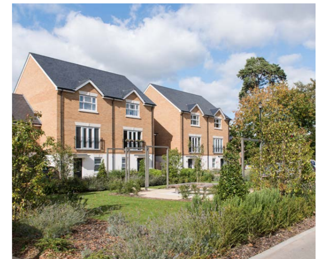
Fig 12: Wates Developments Joint-Ventures
