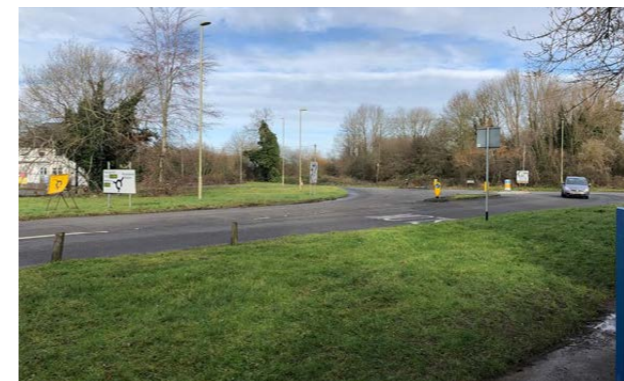
Fig 14: View of existing roundabout between the A30 and Oxford Road
