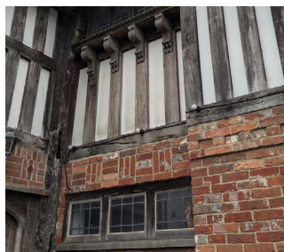
Figure 4.1: Local materials shaping the identity of Bishop's Waltham
