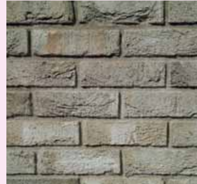
The buff brick used on this scheme on Chilbolton Avenue has a very mellow, almost stone-like colour. It also has a rough finish, resulting in a pronounced and interesting texture.
