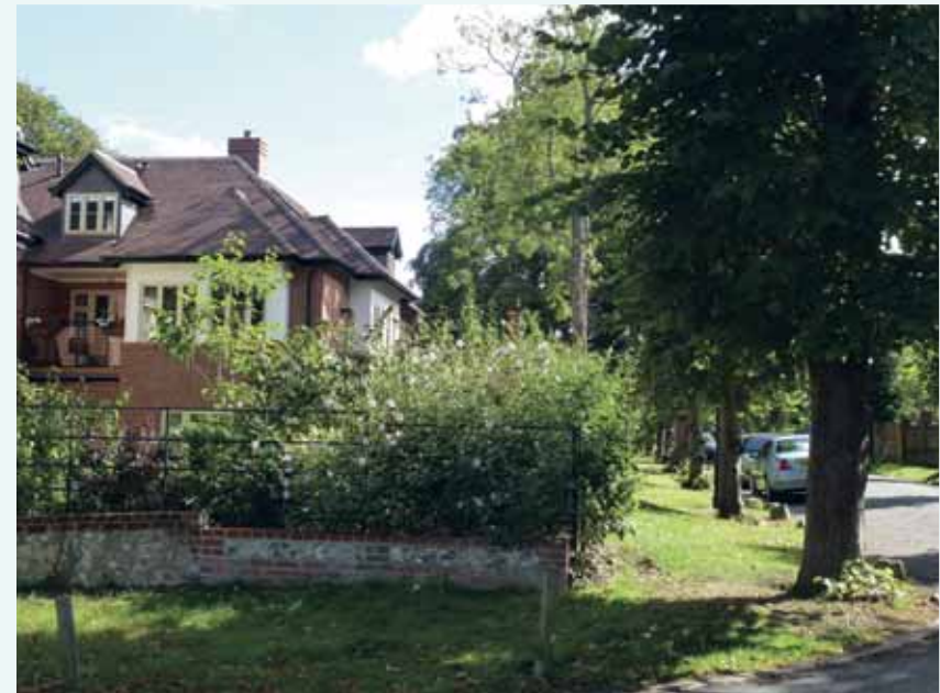
The Milesdown development on St Giles Hill is an example of a successful relationship between the buildings and landscape design.
