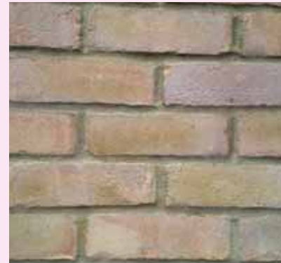
This mellow stock brick (Leicester Multi Stock) used on the Queens Road student accommodation is very subtle and successful, and works harmoniously with grey materials such as Zinc.
