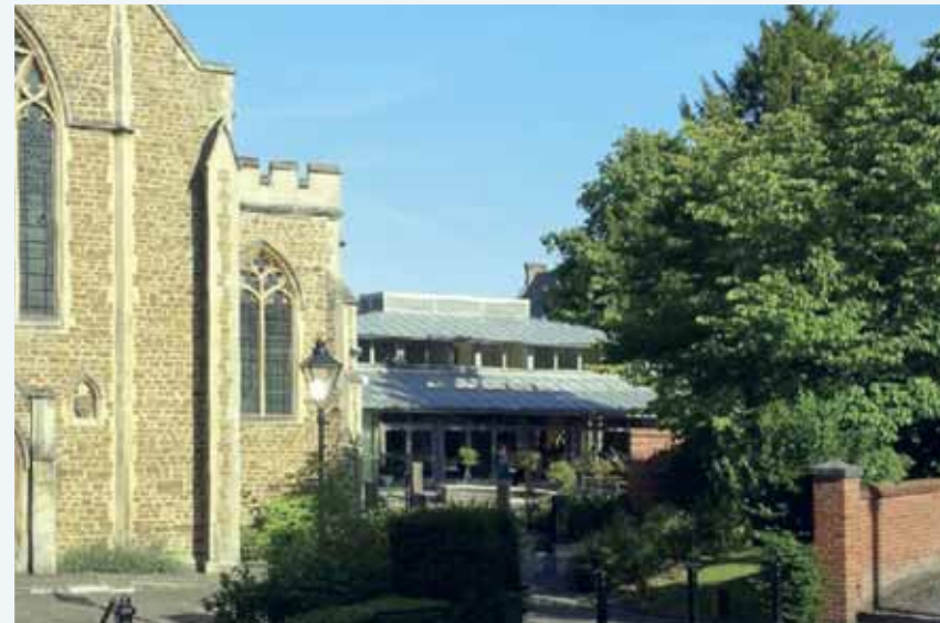
This extension to St Peter's Church in Winchester utilises a modern design, offering a subtle juxtaposition with the listed building, and enhances the character of the area.
