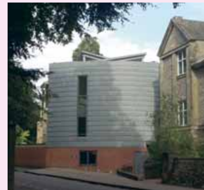
These examples of grey and black zinc give a good idea of the versatility of the material. The colour tone can also work effectively with more traditional materials.
