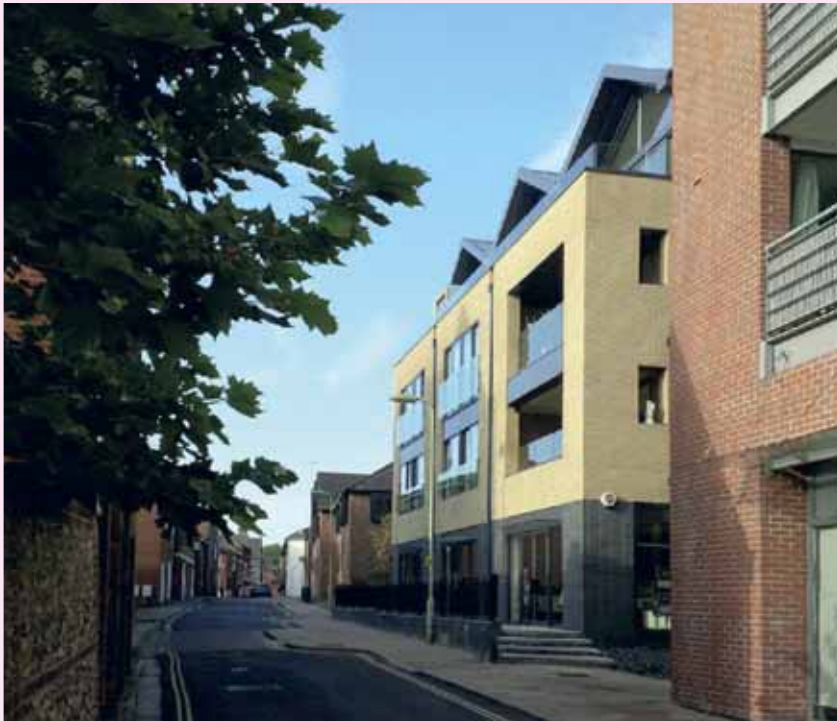
This building on Staple Gardens utilises a buff brick with a very mellow colour tone, allowing for successful integration into the street scene.
