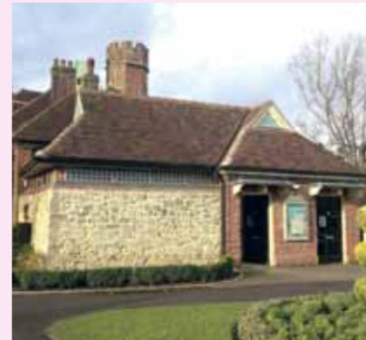
Examples of clay plain tiles, with colour tones ranging from warm orange to dark brown. In both cases the tiles have a traditional, textured appearance.
