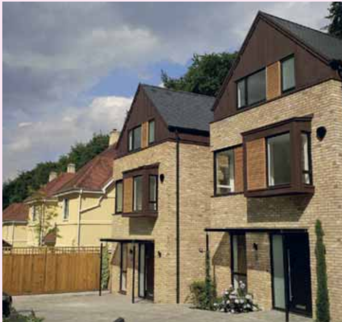
This scheme on Chilbolton Avenue utilises high quality, durable window and door frames (powder coated aluminium) in a colour that contrasts with the buff brick
