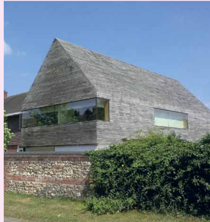
This timber cladding used on a building in Longstock in the Test Valley has weathered gracefully to silver, resulting in subtle gradations of colour.
