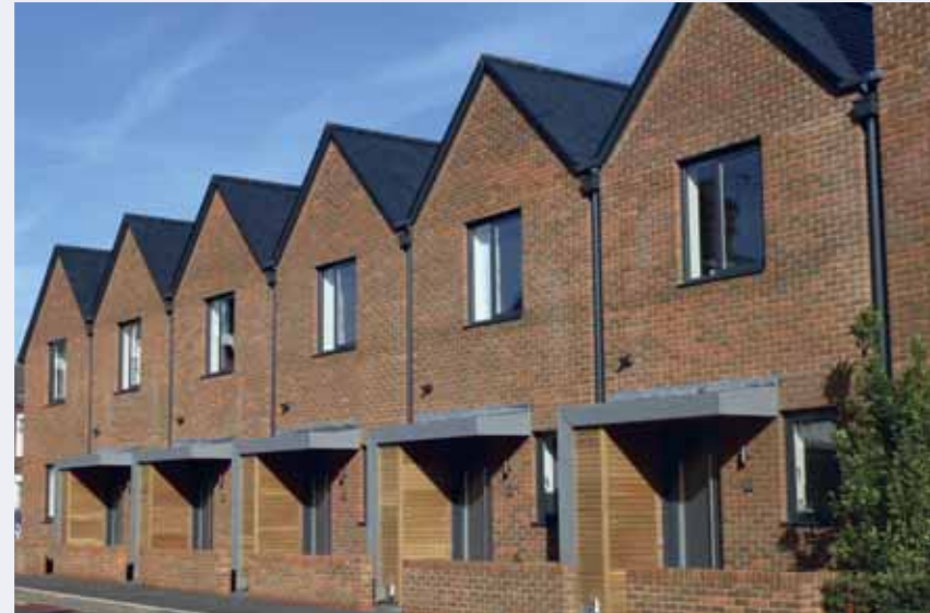
This development utilising a traditional form with a contemporary language responds positively to the terraced typology of Hyde.
