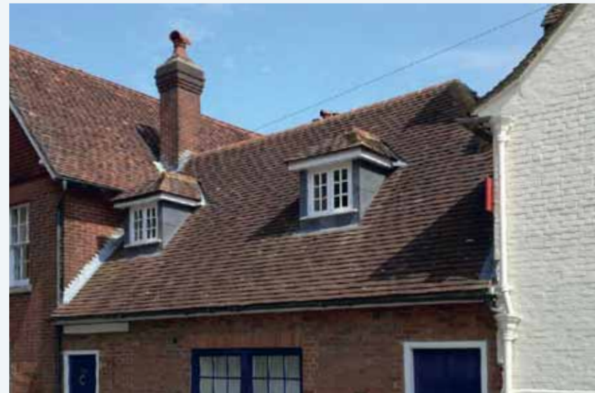
These dormers utilise excellent materials and detailing, and the scale and proportions relate successfully to the existing roof.
