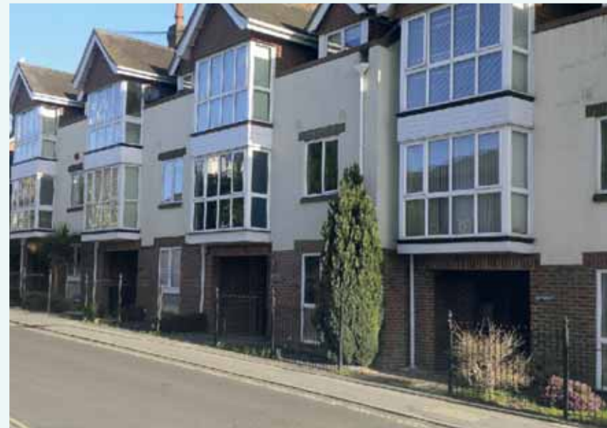
This is a good example of undercroft parking. The parking spaces have a minimal visual impact on the overall composition and the street scene.
