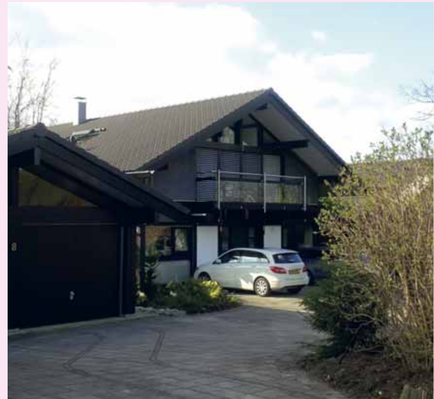
Huf houses are an example of sustainable design, e.g. through the prefabricated construction process and high levels of insulation.
