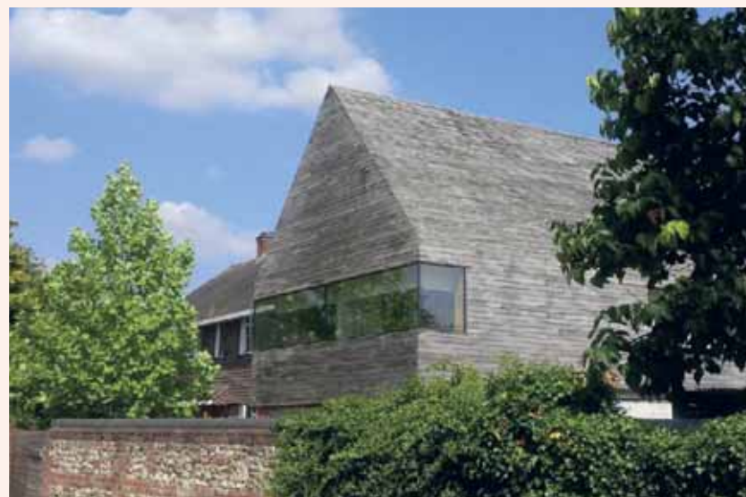
This building in Longstock in the Test Valley reinterprets the traditional rural roof form in a contemporary manner, creating a distinctive shape, reinforced by secret gutters.
