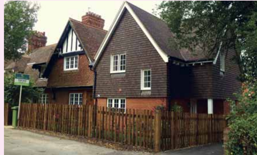
High quality traditional materials and detailing in Micheldever Station, with open eaves, recessed windows and textured clay tiles.
