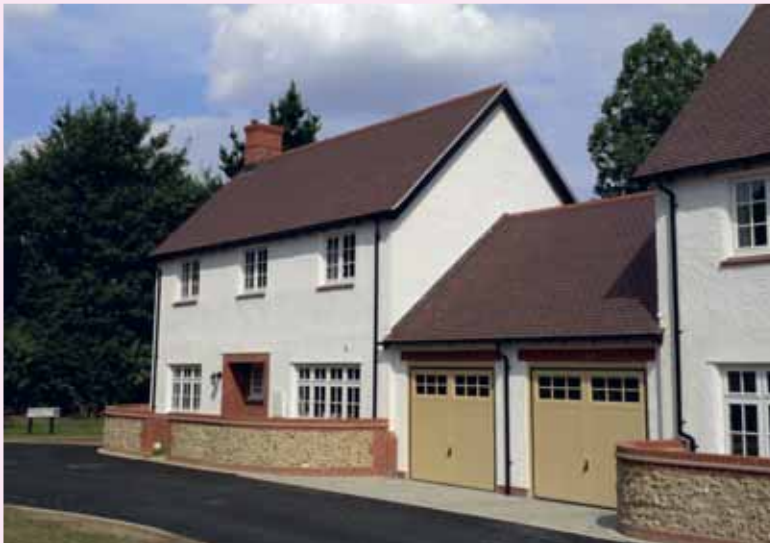
The Francis Gardens site in Winchester utilises rough render, giving an attractive traditional appearance.
