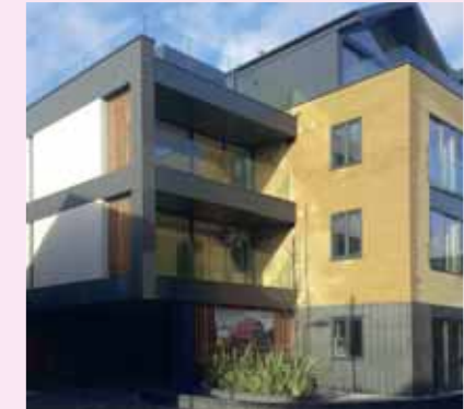
Fibre cement cladding can offer a crisp, interesting appearance (left). The white cladding on the right is a porcelain cladding, with a precise, crisp finish.
