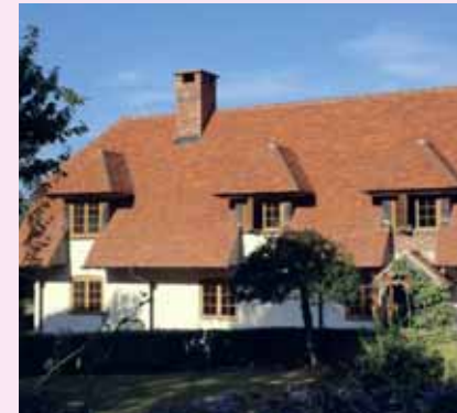
Examples of clay plain tiles, with colour tones ranging from warm orange to dark brown. In both cases the tiles have a traditional, textured appearance.
