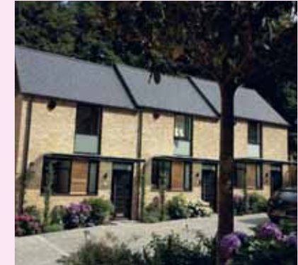
The buff brick used on this scheme on Chilbolton Avenue has a very mellow, almost stone-like colour. It also has a rough finish, resulting in a pronounced and interesting texture.
