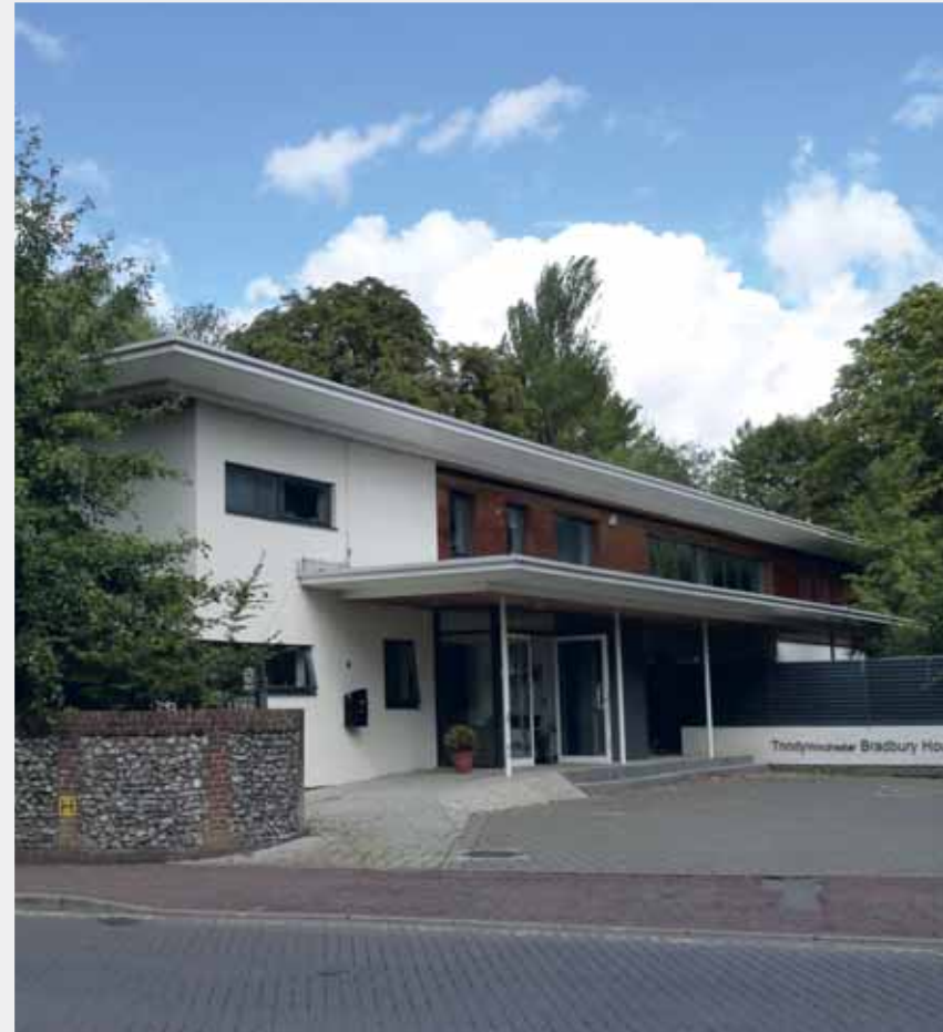
A crisp contemporary design at Durngate, Winchester.
