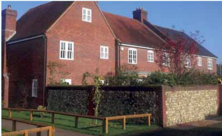
In this example in East Meon the boundary treatment has been designed in such a manner as to complement the overall design concept for the site and the local context.
