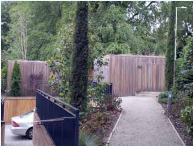
Well designed bin and cycle storage at the former Ambulance Station site, Winchester.
