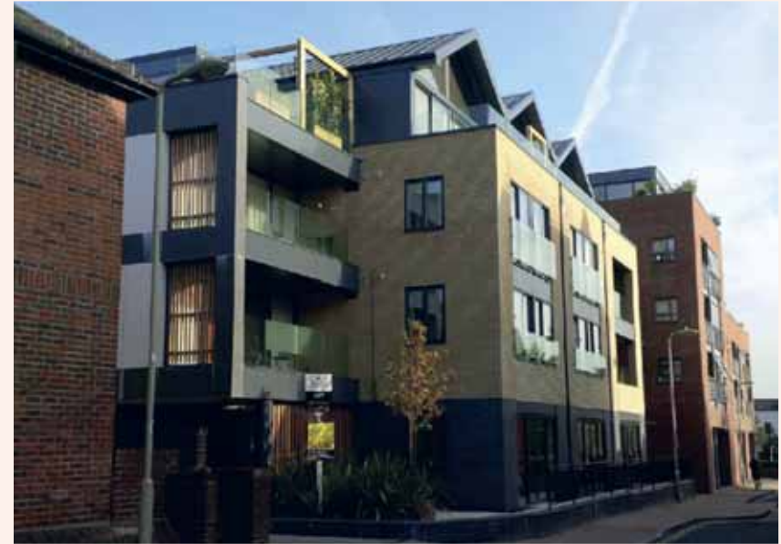
The set back top storey in this example incorporates a pitched roof form, which has been carefully designed to give the building rhythm and an elegant meeting with the sky.
