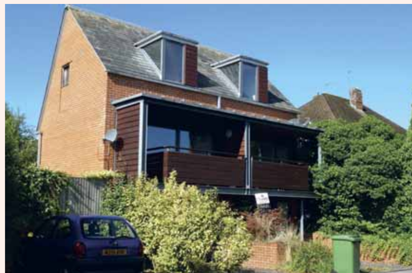
These dormers positively reinforce the overall design ethos, with their contemporary character, and crisp, detailing and good quality materials.
