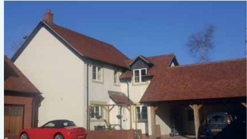
In this example from Hambledon the parking has been provided to the side of the buildings, which reduces its impact on the public realm. The car port has also been designed in a high quality traditional manner, to complement the overall design ethos for the development.
