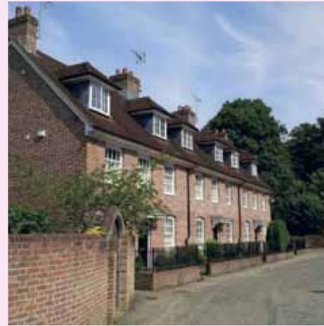
An example of robust metal railings combined with brickwork. This suits the design of the houses.
