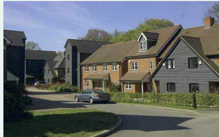
These connected dwellings at Micheldever Station define and enclose the public realm.
