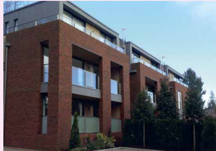
This development in Winchester utilises high quality stock bricks, well detailed balconies and a subtle blend of traditional and contemporary materials.
