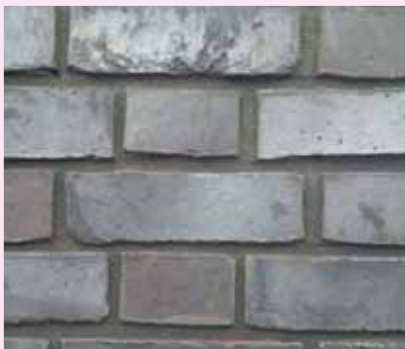
Successful use of dark bricks and colour matched mortar in Winchester.
