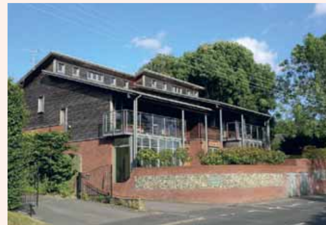
The balconies on this building in Kings Worthy enliven the frontage and ensure the building engages with the public realm.
