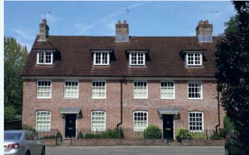
This excellent development in Twyford utilises a high quality courtyard. The design of the courtyard reinforces the sense of place.
