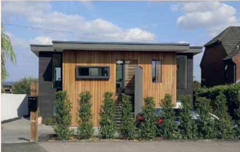
This example employs a contemporary approach to the fenestration in terms of shape, size, arrangement, materials and detailing.
