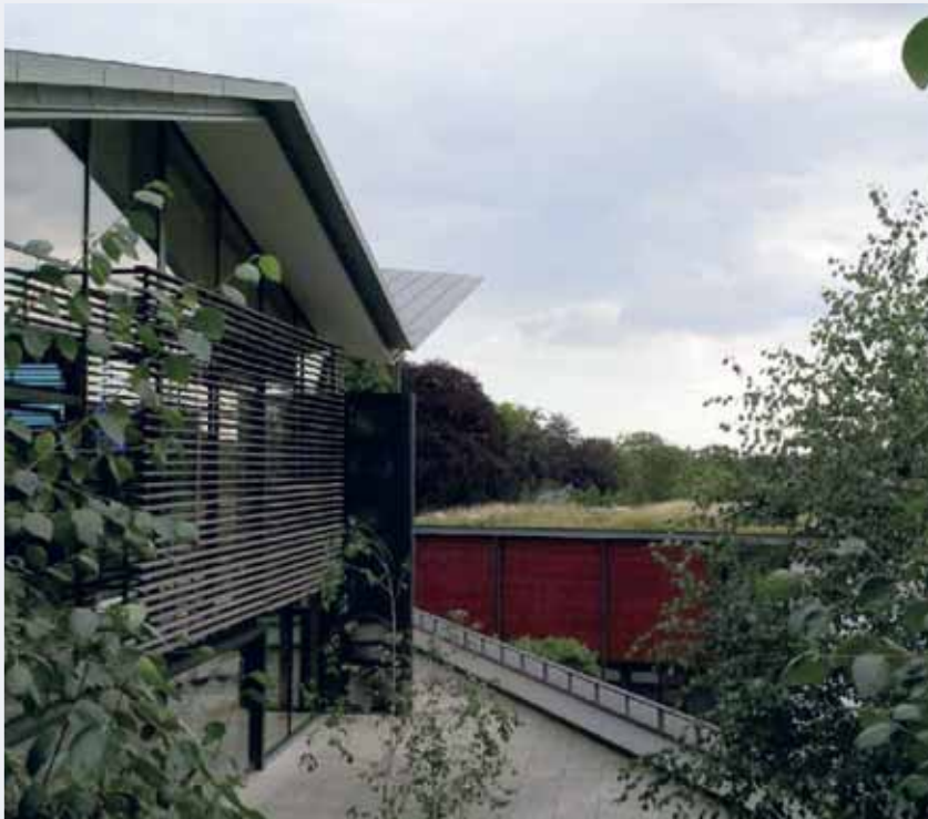
Good example of sustainable design at Winchester University, including triple glazing, louvers and a green roof.
