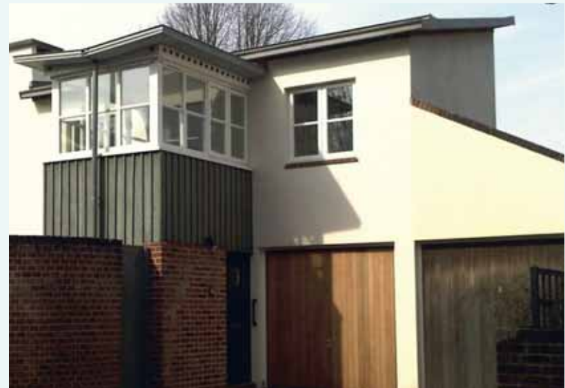
This is an example of the successful incorporation of integral garages in Winchester. The garage doors do not dominate and fit well with the design of the buildings and boundaries.
