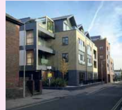
This example in Winchester illustrates the benefits of dark bricks, and how the positive effects are accentuated by the use of colour matched mortar, and an interesting brick bond, in this case stack bond.
