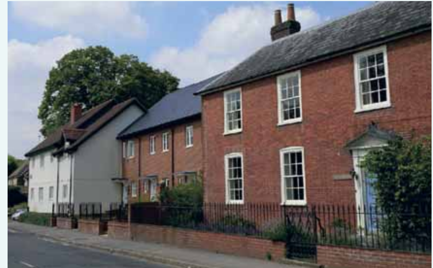
In this example from Hambledon the new development accords with the locally distinctive form of defining the front boundary.
