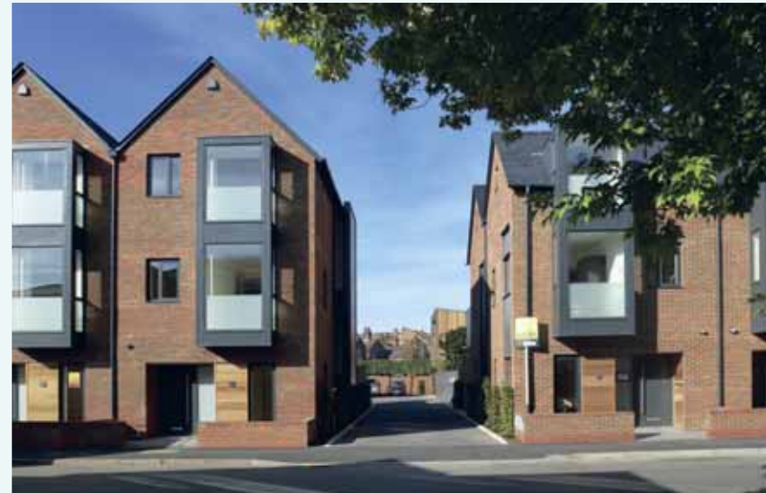
This rear access road has been softened with planting, whilst the parking area also benefits from planting in the form of pleached trees. The hard surface has been designed to demarcate the parking spaces. The parking area is also well-overlooked (see image on page 44 for a view from the rear parking area).
