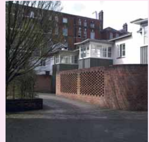
This example in Winchester uses high quality brick walling, laid with an interesting brick bond to create visual interest and defused views into and out from the gardens.
