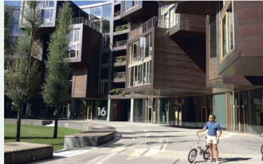
This development in Copenhagen (Tietgen Dormitories) demonstrates the significant effect of shape on the quality of spaces, creating enclosure, enriching the pedestrian experience, providing an intimate and dramatic space.
