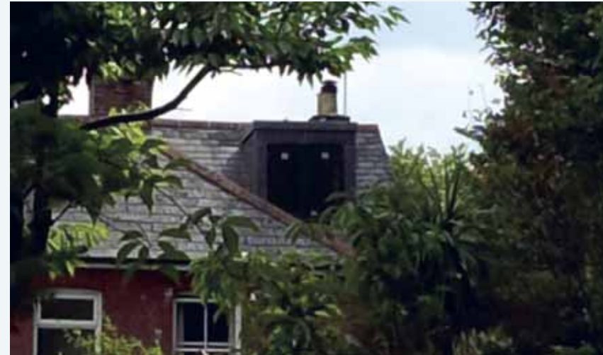
This dormer window in Hyde is well related to the existing property in terms of scale. The use of dark grey materials provides a successful visual relationship with the existing slate roof.
