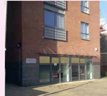
In this example, the lack of colour matched mortar perhaps undermines the appearance of the dark bricks, and the combination with red brick is also not as successful.
