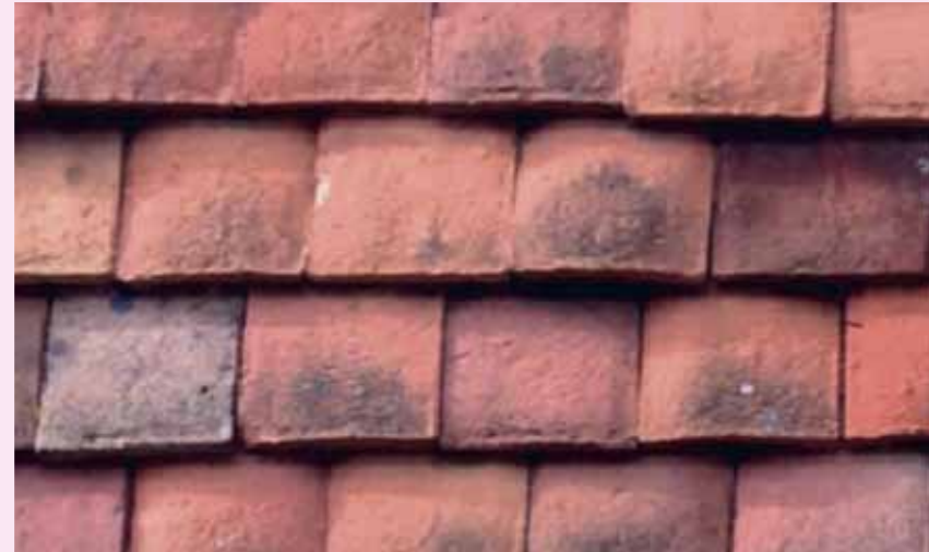
Examples of good quality plain clay tiles, note the colour tones, shape and texture of the tiles (image from Barton Farm Design Code).
