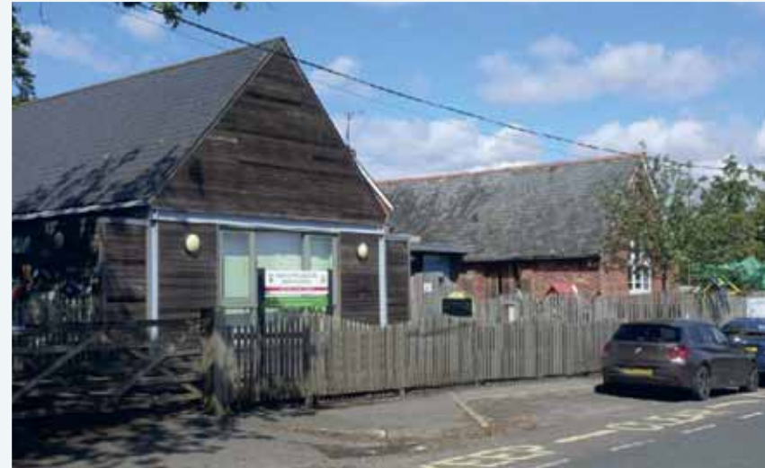
This extension near Newtown has been sensitively located to the host building in terms of alignment form and scale, with the contrasting material reflecting the transition of the building form.
