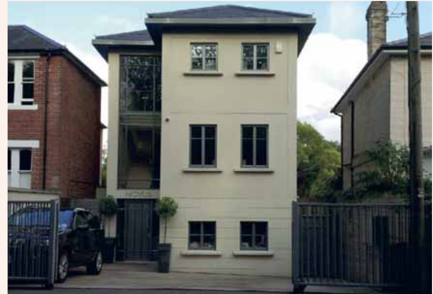
The proportions of the front elevation are slender and elegant. The arrangement of windows using different sizes in an ordered way, reinforce that impression.
