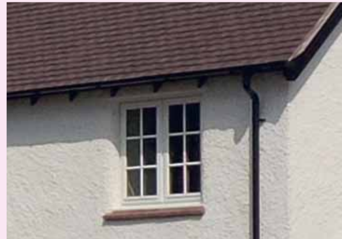
Successful traditional eave detailing; note the benefits of the dark, open eaves and barge boards.
