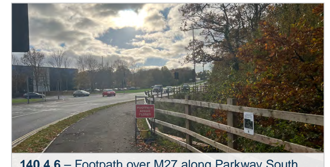
140.4.6 – Footpath over M27 along Parkway South roundabout
