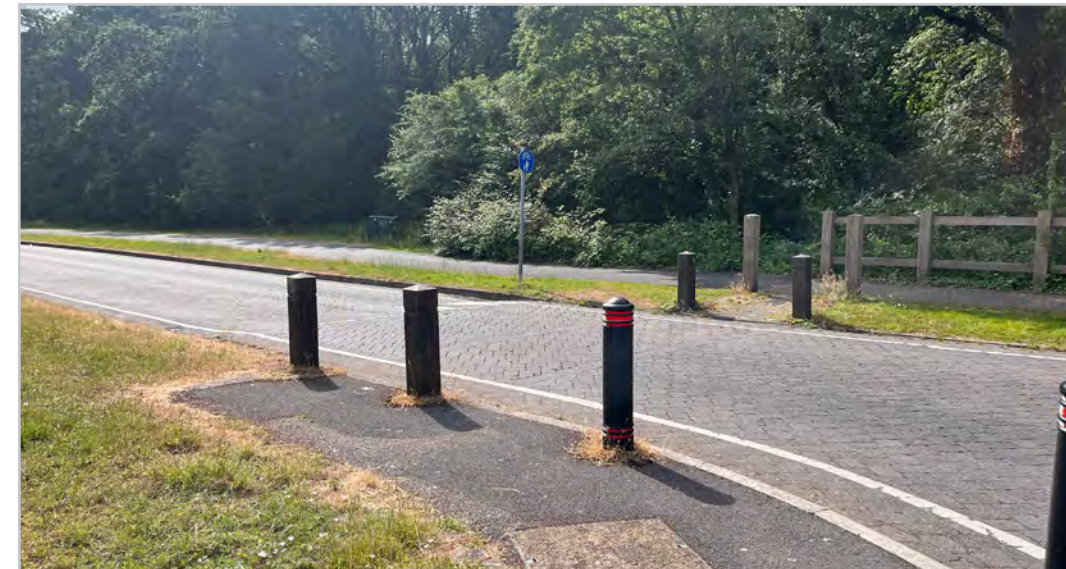
Z3.1.4 – Bollards at junctions along Marjoram Way
