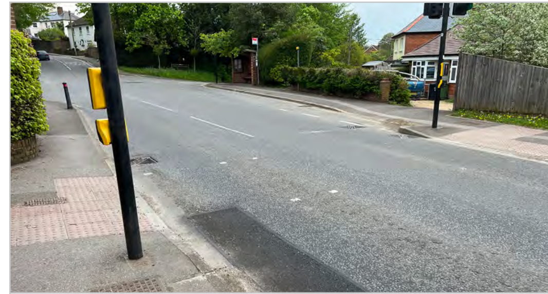
130.1.6 – High Street/Hazeley Road junction
