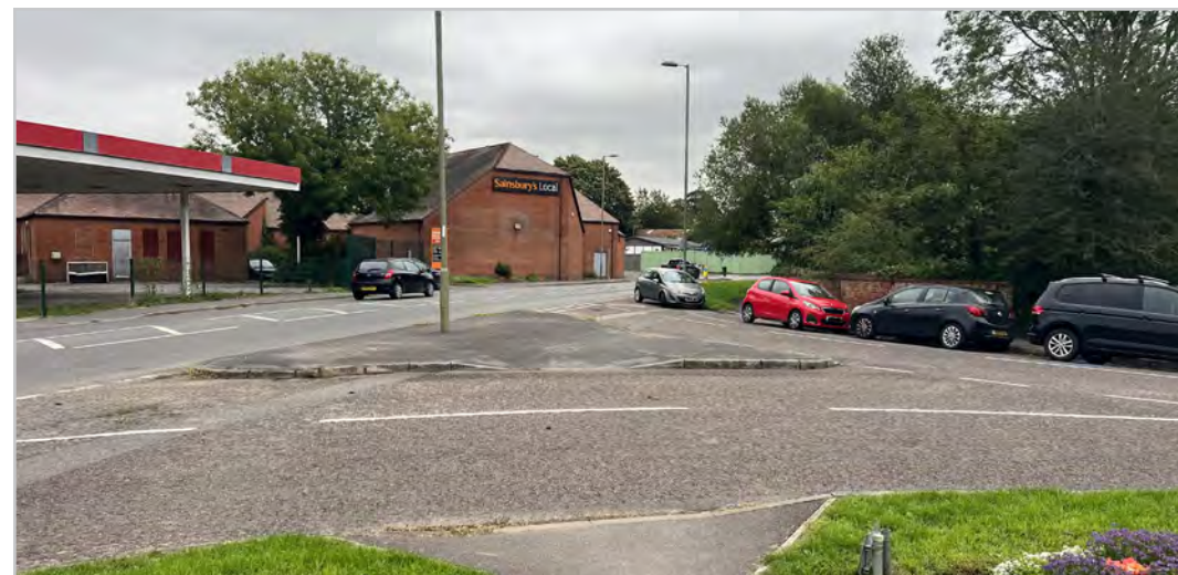
Z2.2.2 – B2177/Station Road junction/Bishop's Waltham Palace
