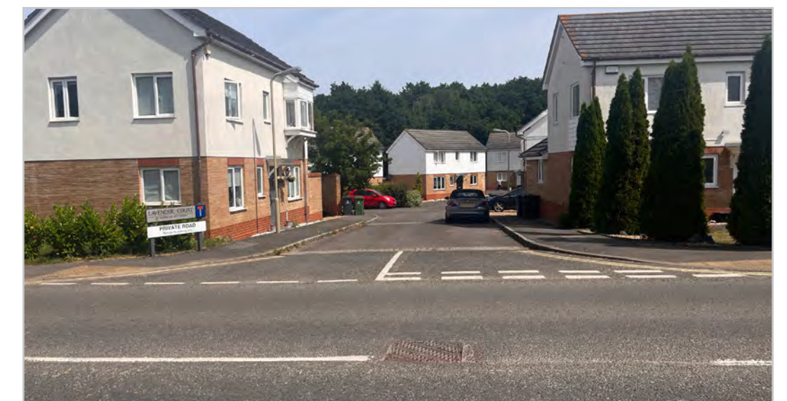
Z3.5.5 – Bluebell Way/Lavender Court junction
