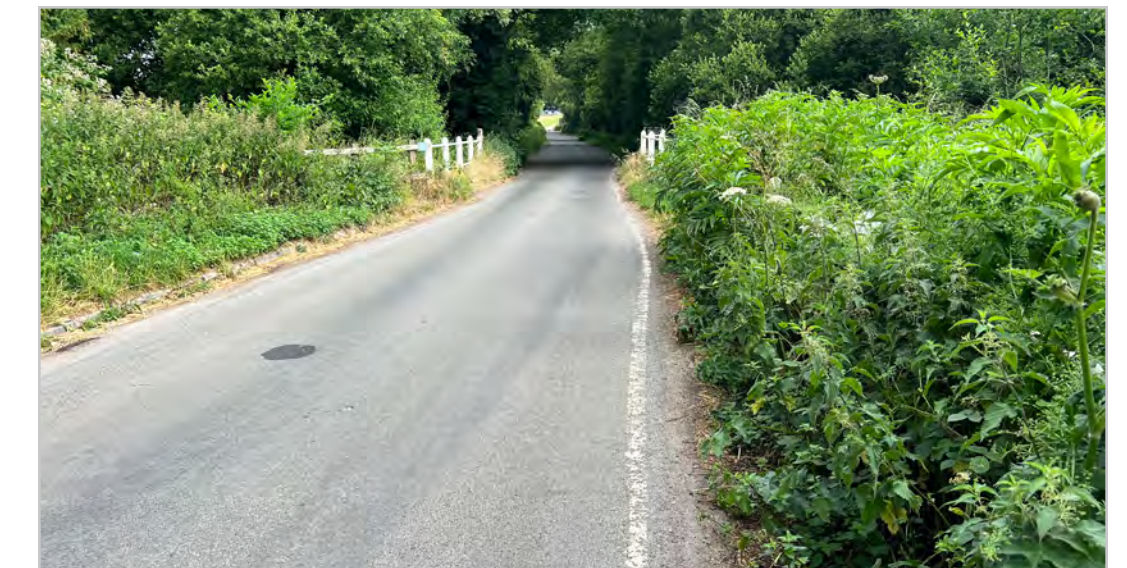
100.1.2 – Bridges along Easton Lane
