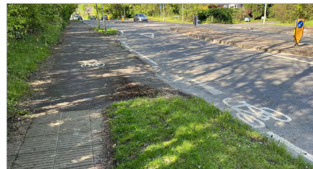
120.1.7 – Main Road/Poles Lane roundabout
