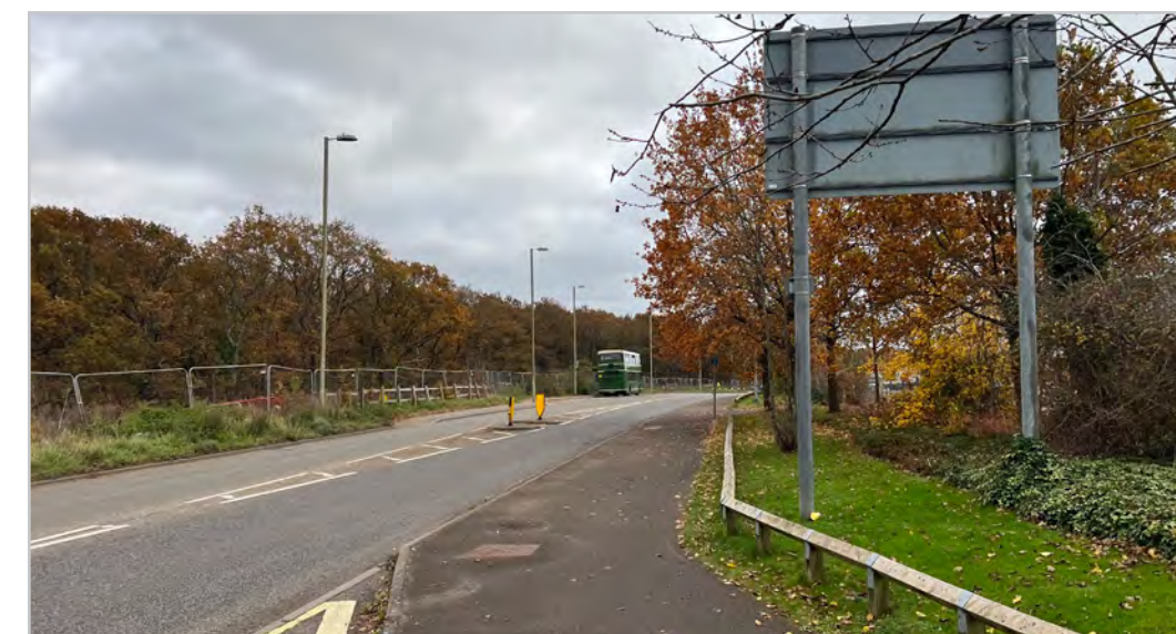
140.4.2 – Whiteley Way along Whiteley village
