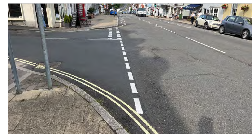
Z1.1.4 – West Street/Station Road junction
