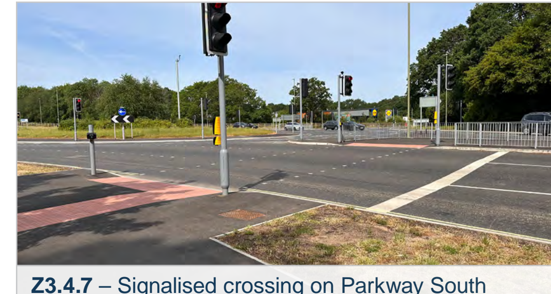
Z3.4.7 – Signalised crossing on Parkway South roundabout
