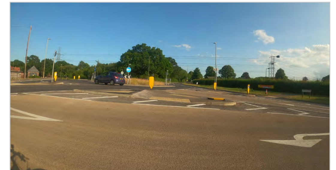
130.5.4 – School Road/Hoad's Hill roundabout
