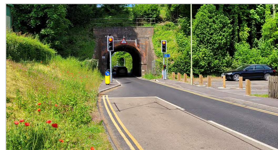
200.2.5 – Wellhouse Lane underbridge
