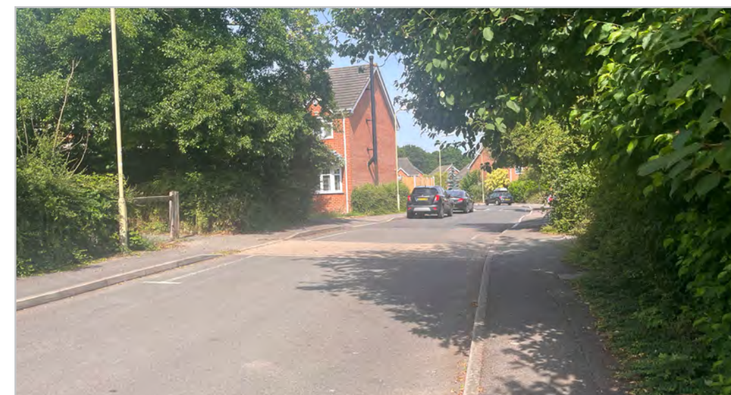
Z3.2.3 – Footpath crossing Saffron Way
