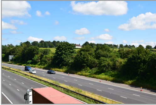
North-east towards Alresford Road from footbridge over M3
