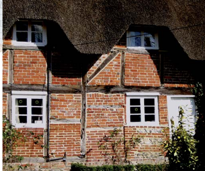
6 & 7 Mill Lane timber frame with brick infill
