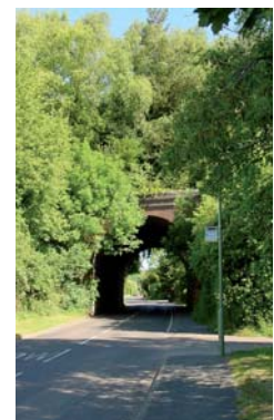
Springvale Road railway embankment
