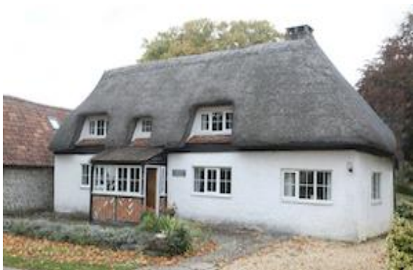
Figure 16: Conservation Area Building (2020).
