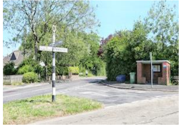
Figure 27: Pedestrian Risk Area 2 Main Road/Kennel Road crossroads (2020).
