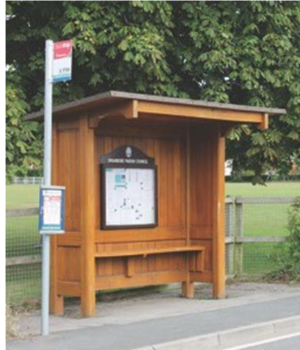
Bus shelters have been installed where pavements are wide enough.
