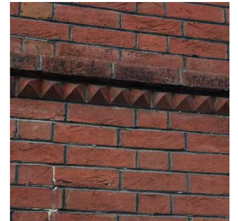
Brick Feature Detailing
