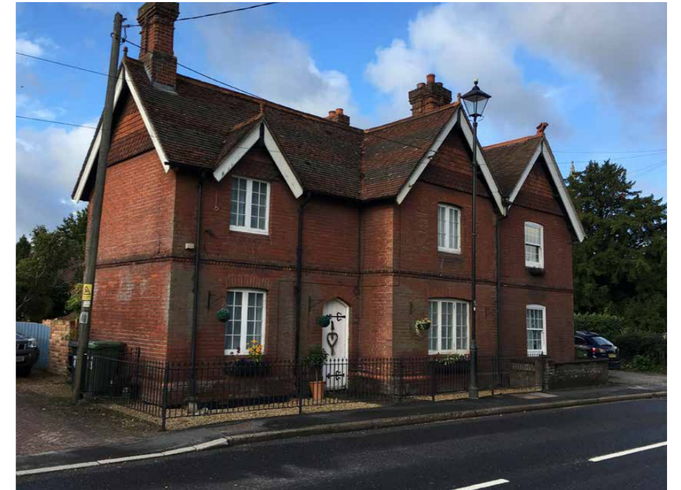
Semi-detached house with double front gable detail, tile hanging to gables, arched brick headers, and dogtooth course brick detail.
