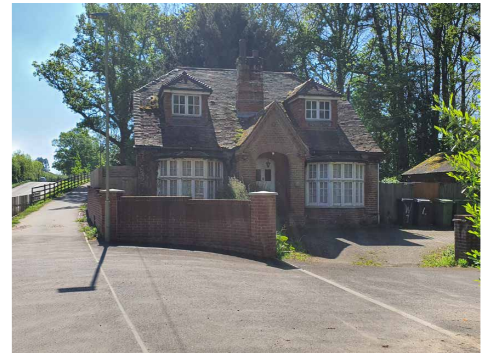
Detached Chalet Bungalow with built-out gable porch and symmetrical ground floor bays on A3051, opposite the southern end of Outlands Lane.
