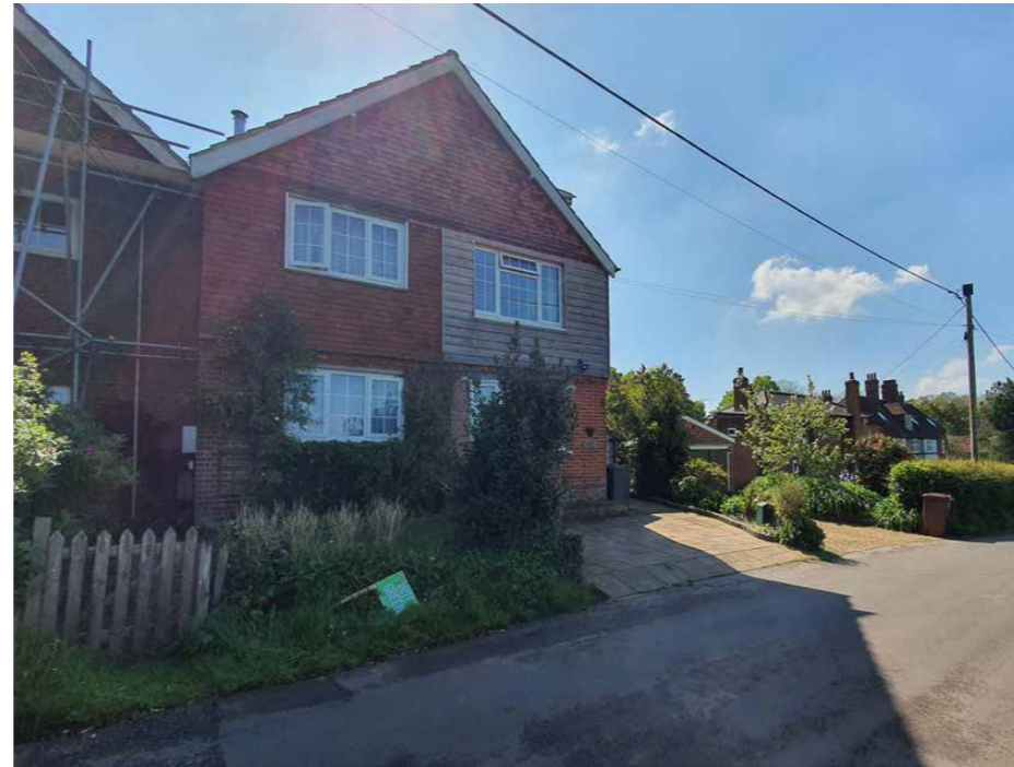
Semi-Detached House with both tile hanging and timber boarding to the front facade.
