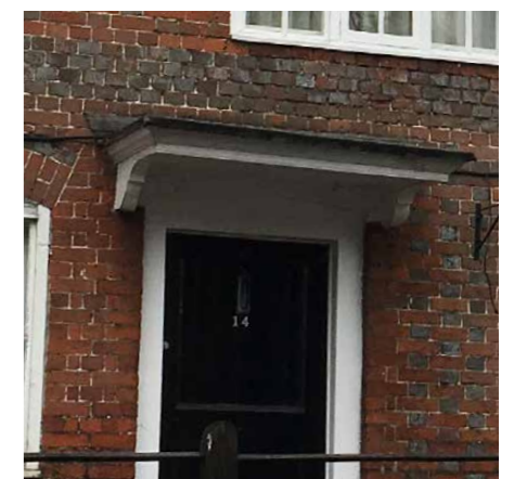
Flat-roofed Canopies to Front Doors
