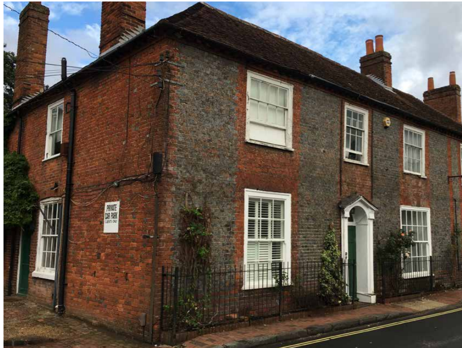
Georgian house with grey brick front facade, burnt-end brick side façades, skewback arch brick headers, and larger windows to ground floor.
