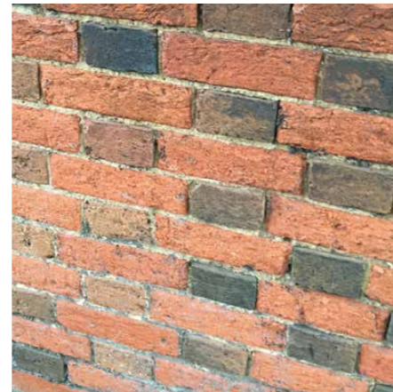
Flemish Bond in Burnt-End Brick
