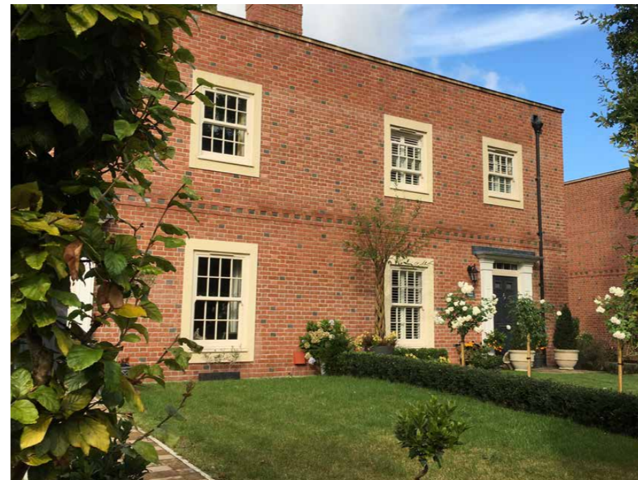
Georgian-Style Houses with parapet roof, dentil course brick detail, and stone-effect window surrounds.
