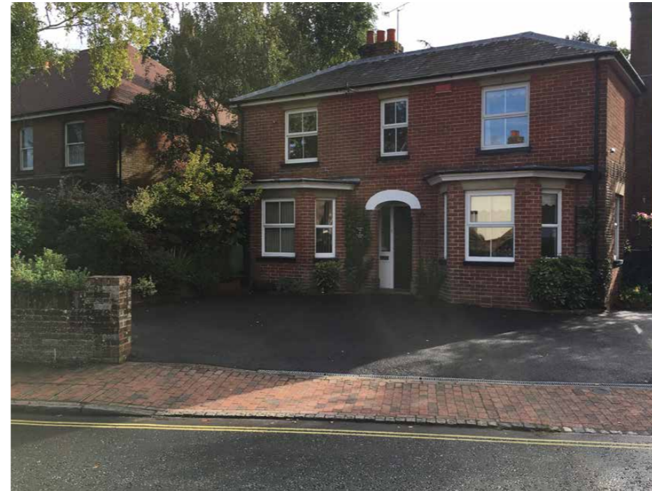
Detached house with recessed porch, symmetrical ground floor bay windows, and skewback arch stone headers.
