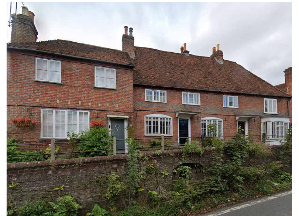
Historic Terraced Housing on Mill Hill/A334
