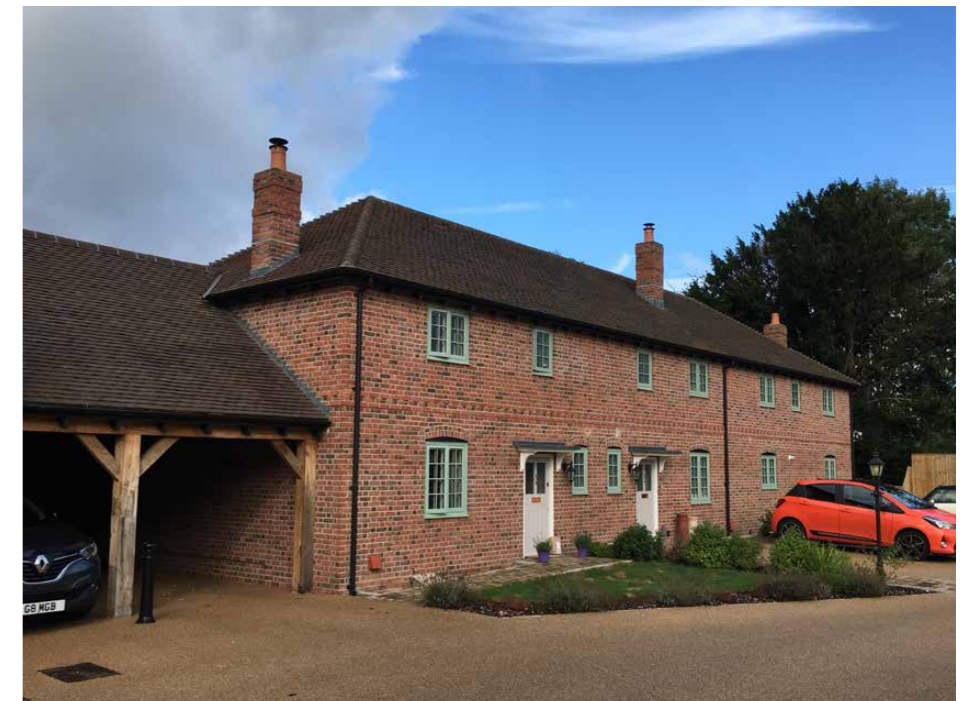
Farmyard-Style Terraced Houses with dentil course brick detail, chimneys, and flat canopies to front doors.
