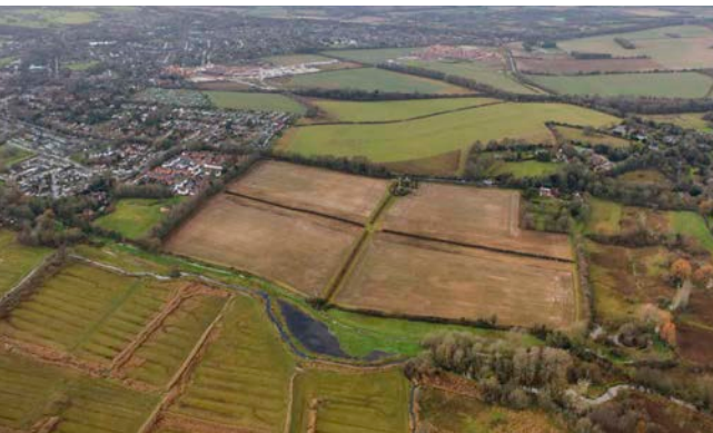
View looking west across the site with the Kings Barton/Barton Farm development in the background
