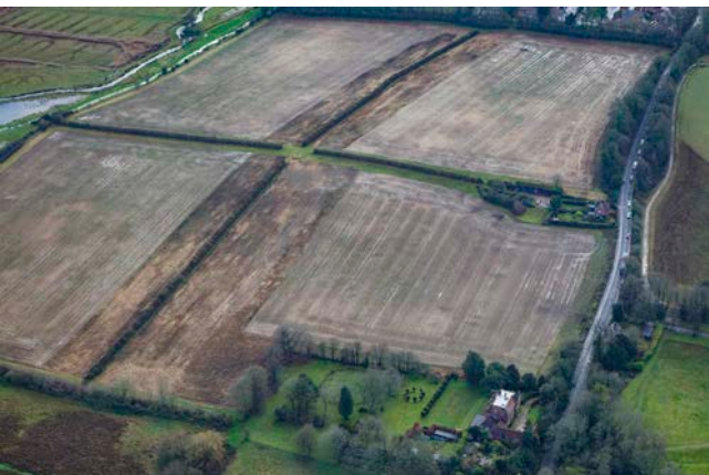
Close up view of the site looking south with the cottages of Worthy Road/London Road in the foreground
