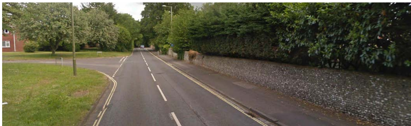
Footway on Worth Road into Winchester city centre
