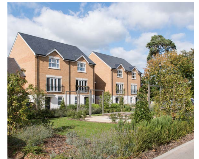
Fig 12: Wates Developments Joint-Ventures
